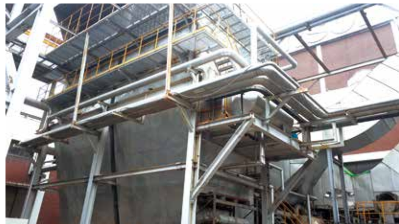
Hansol HomeDeco Iksan Plant Waste Heat Recovery System
