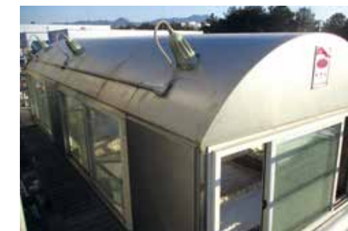
Hansol Chemical Dissolved Air Flotation Tank
